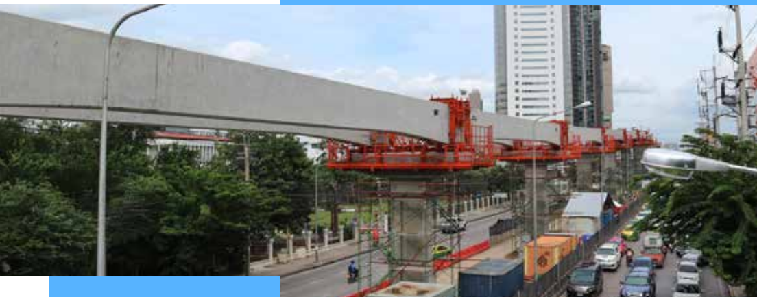
Construction of monorail line in Bangkok (photo courtesy of BTS Group).
